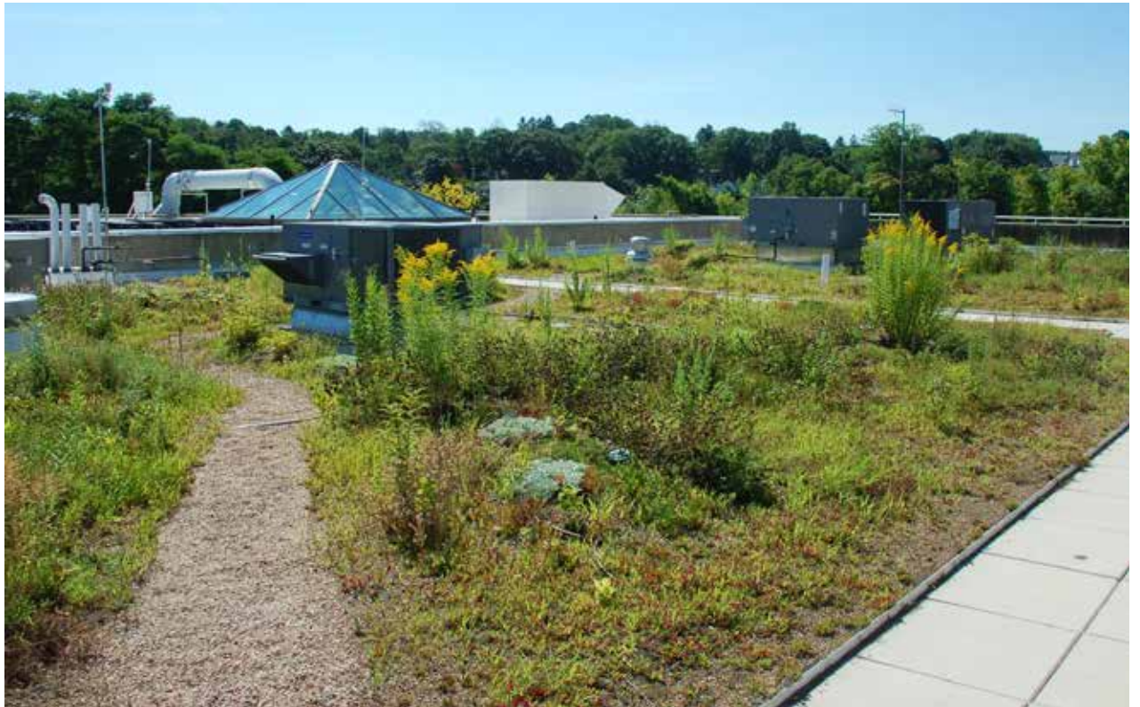
Completed in 2011, the showcase green roof at the Lowell Regional Wastewater Utility measures roughly 6,300 square feet and has dramatically reduced stormwater runoff at the treatment plant.
